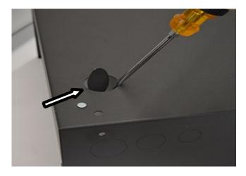
8. Remove the knock out on the back of the enclosure.
